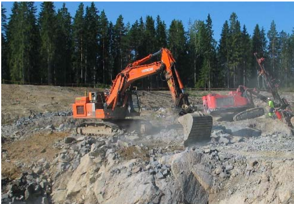
Waste stripping at Kujankallio Open Pit
